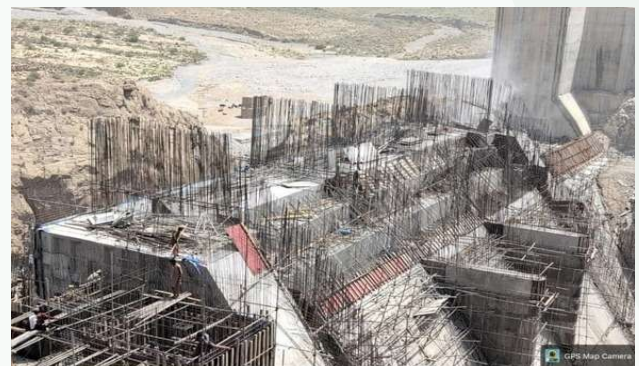
Downstream view Mangi Dam
