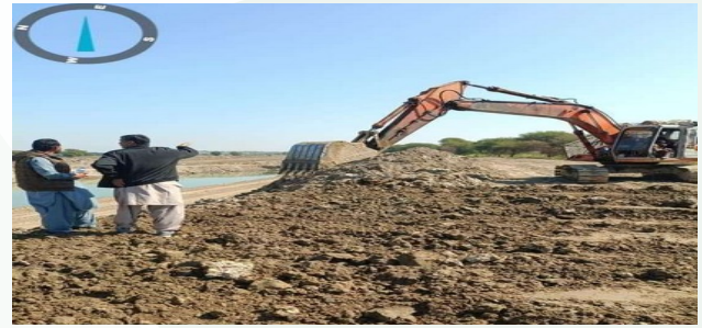
Excavation Work in progress
