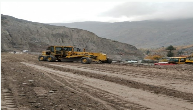
Preparation of Subgrade in Progress
