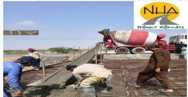
Concrete pouring of top slab of culvert
