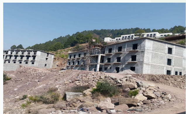
Administration Block under Construction
