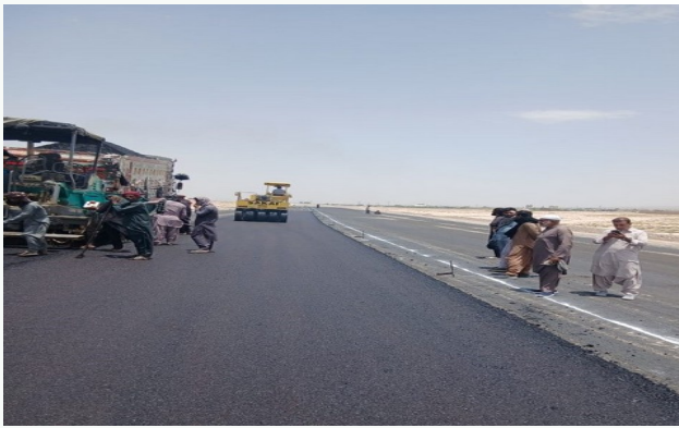
Compaction of Asphaltic wearing course
