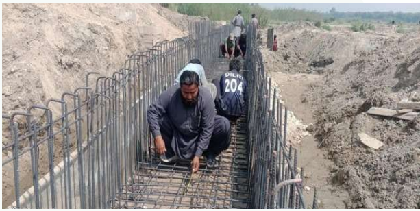
Steel Fabrication for Watercourse
