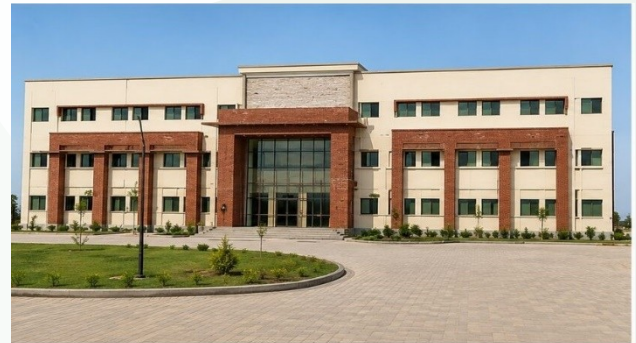
Girls Hostel Construction under Progress
