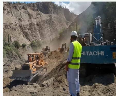
Slope Cutting in Progress
