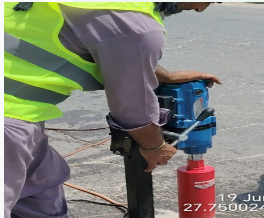
Core Cutting in Progress
