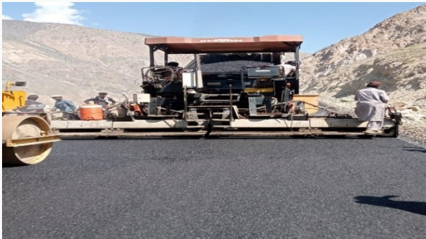
Laying and Compaction of Asphalt
