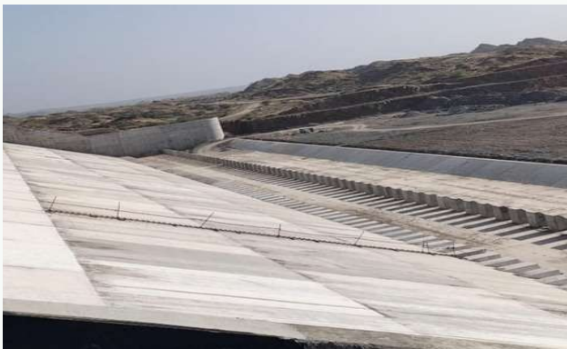
View of Stilling basin, Baffle block Spillway
