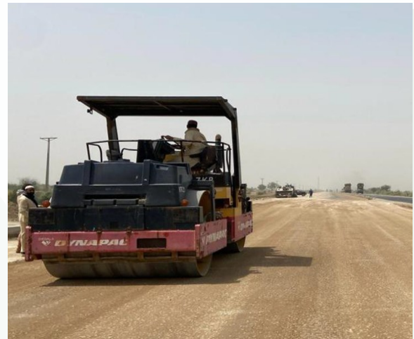
Compaction of Aggregate Base Course
