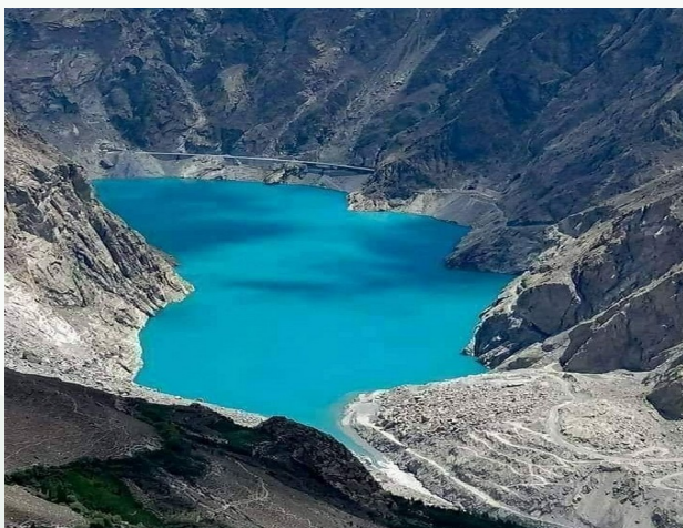
Attabad Hydropower Project Site
