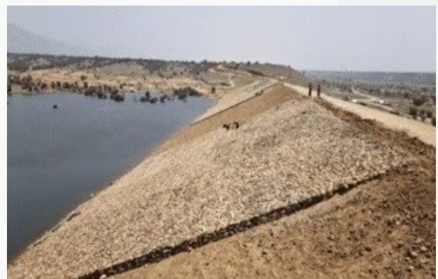
Protection Works at DUB Dam
