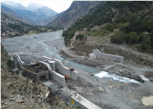
Lawi Hydropower Project – Weir / Intake
