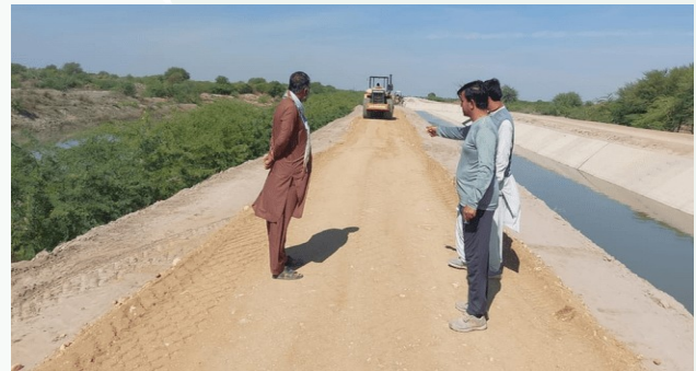
Compaction of Sub-grade by Vibratory Roller Between RD 76 and 90
