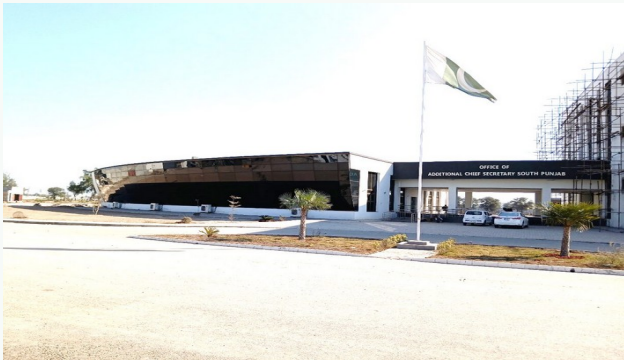
Main Building (Zone-6)
