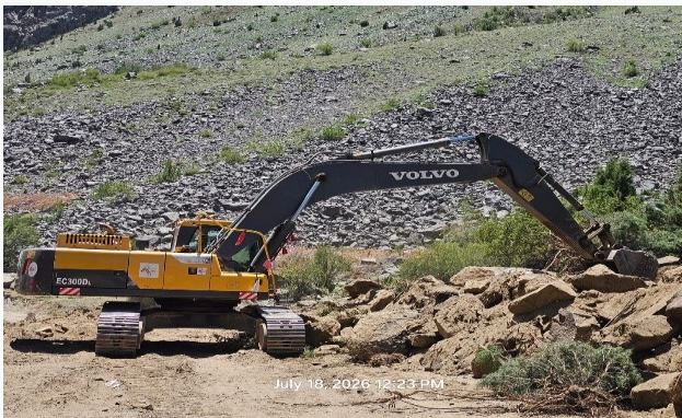
Clearance of Rock debris
